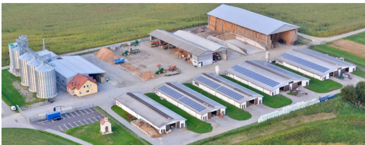
Figure 28: Farm ŽIPO Lenart with barns for cattle and fodder storage facilities.
